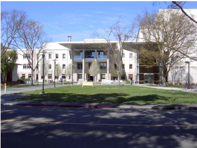
Exterior of the Plant and Environmental Sciences Lab
